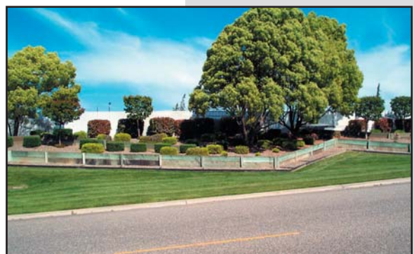
THIS LANDSCAPE BUFFER HELPS TO SCREEN THE PARKING AND LOADING AREAS OF THIS BUILDING.
