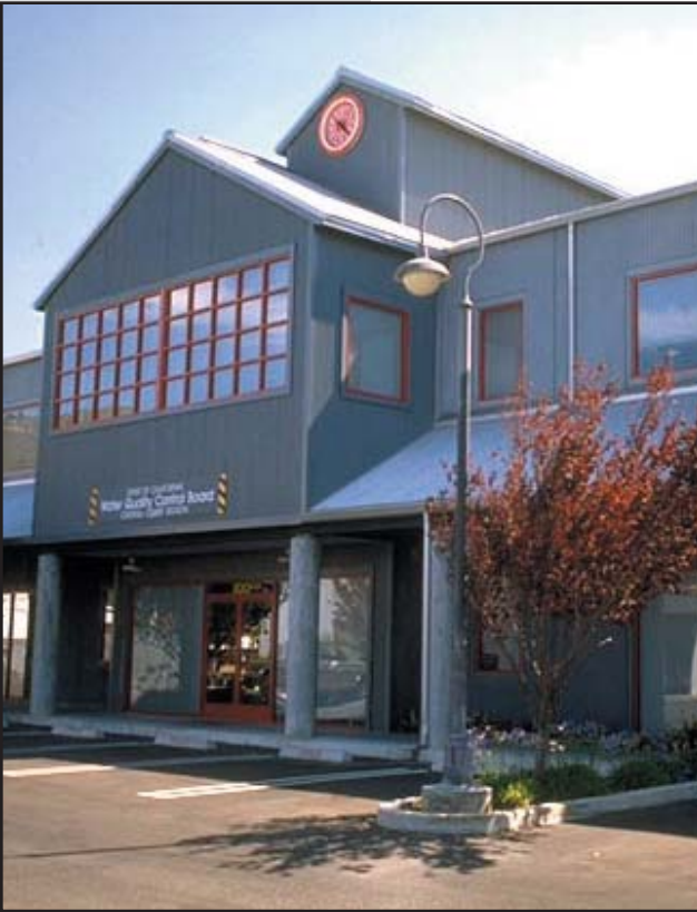
LIGHT FIXTURES SHALL BE DESIGNED OR SELECTED TO BE ARCHITECTURALLY COMPATIBLE WITH THE MAIN STRUCTURE OR THEME OF THE BUILDING.
