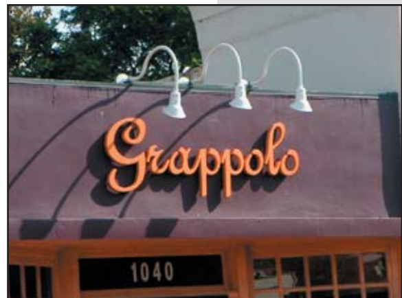
SIGNS SHALL BE ILLUMINATED EXTERNALLY WITHOUT PRODUCING GLARE ON PEDESTRIANS, AUTOS, OR MIXED-USE RESIDENTIAL UNITS.
