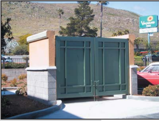
TRASH ENCLOSURES SHALL BE DESIGNED WITH MATERIALS AND COLORS THAT ARE CONSISTENT WITH THE ADJACENT STRUCTURE.
