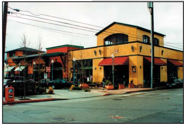
THE COLOR OF AWNINGS AND OVERHANGS SHALL BE INTEGRATED INTO THE OVERALL COLOR SCHEME OF THE PROJECT.
