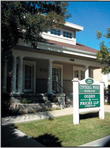
MONUMENT SIGNS THAT USE SIMILAR COLORS AND MATERIALS AS THE MAIN BUILDING, SUCH AS THIS, ARE APPROPRIATE FOR RESIDENTIAL/OFFICE CONVERSIONS.
