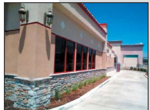
ATTRACTIVE BUILDING FACADES HAVE VARYING TEXTURES, COLORS, AND WALL PLANES.
