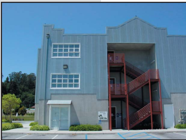
PARAPETS HELP TO GIVE FORM TO THIS BUILDING. IN ADDITION, THE STAIRWELL IS INTEGRATED NICELY AND PROVIDES RELIEF INTO THE BUILDING FACADE.
