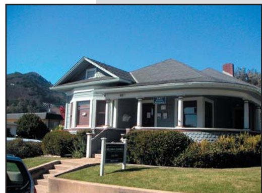
BY RAISING THE FOUNDATION, THIS BUILDING APPEARS TO BE IN SCALE WITH LARGER ADJACENT BUILDINGS.
