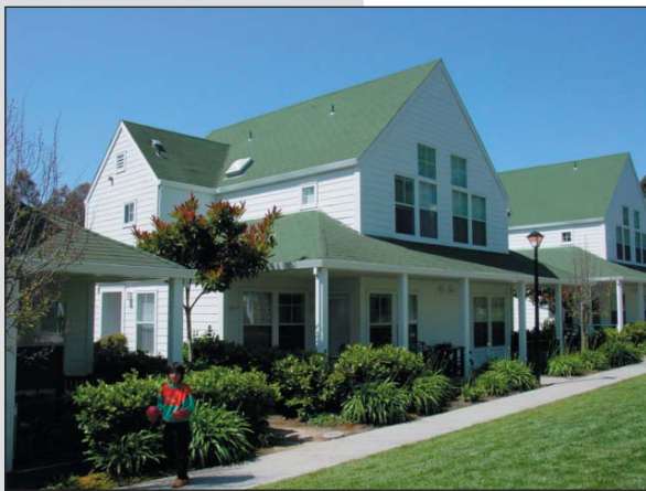
BUILDING MASS CAN BE BROKEN UP WITH VARIOUS ROOF FORMS AND THE ADDITION OF PORCHES.
