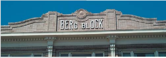
BUILDING PARAPETS AND CORNICES GIVE IDENTITY TO A BUILDING AND HELP TO SCREEN ROOFTOP EQUIPMENT.
