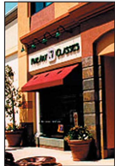
AWNINGS SHALL BE MADE OF CLOTH AND BE PLACED HIGH ENOUGH SO AS NOT TO INHIBIT PEDESTRIANS.
