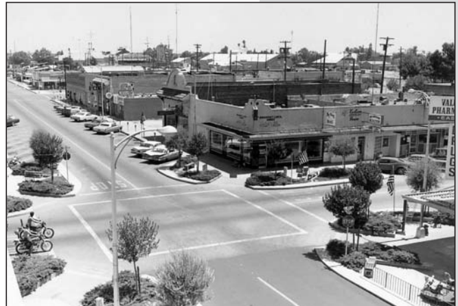
LANDSCAPING AND BULBOUTS MAKE THIS A PEDESTRIAN FRIENDLY INTERSECTION.
