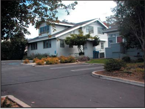
PARKING LOTS SHALL BE LOCATED AT THE REAR OF THE BUILDING OR IN PARKING "COURTS".
