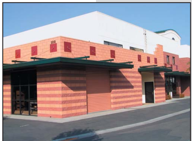
VARIATION OF BUILDING FORMS AND PLANES EMPHASIZE THE ARCHITECTURAL CHARACTER OF THE BUILDING.
