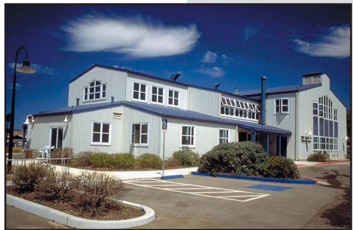
VARIATION IN WALL PLANES HELP TO BREAK UP THE MASS OF THIS BUILDING.
