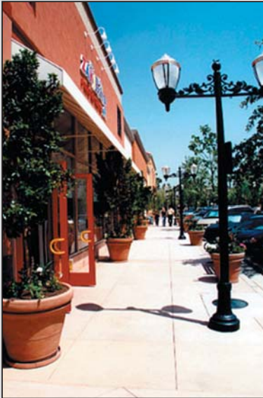
SUBDUED COLORS USUALLY WORK BEST FOR THE OVERALL BUILDING COLOR. ACCENT COLORS SHALL BE USED FOR AWNINGS, DOORS, AND TRIM.
