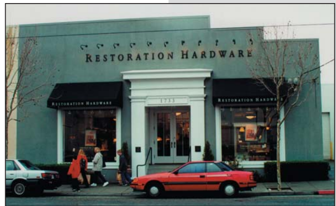
AWNINGS SHALL NOT DOMINATE THE FACADE BUT RATHER BE IN SCALE WITH THE REST OF THE BUILDING.
