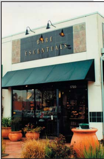
STORE FRONTAGES SHALL INCLUDE AMENITIES SUCH AS TRANSPARENT DISPLAY WINDOWS, MOVEABLE LANDSCAPED CONTAINERS AND POTS AND AWNINGS.
