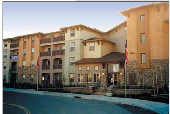
THE USE OF STONE HELPS TO BREAK UP THE VERTICAL MASS OF THE BUILDING.
