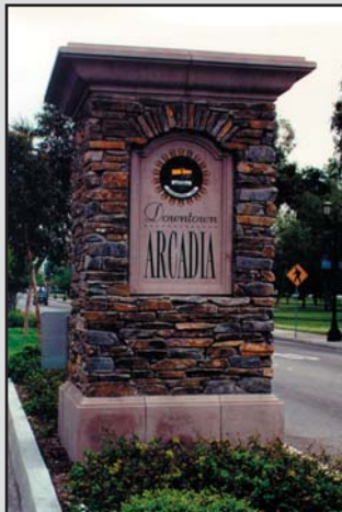
GATEWAY MONUMENTS SHALL BE USED TO ANNOUNCE ENTRY INTO THE DOWNTOWN CORE
