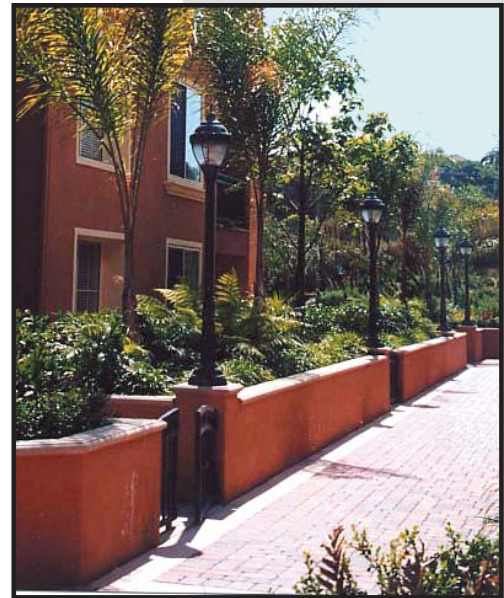
RESIDENTIAL LIGHTING POLES SHALL BE APPROPRIATELY SCALED.
