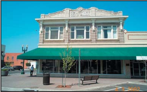
HISTORIC BUILDINGS WITH ELABORATE BUILDING CORNICES HAVE HELPED TO ARCHITECTURALLY DEFINE DOWNTOWN TURLOCK
