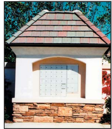
COMMON MAILBOX ENCLOSURES SHALL BE DESIGNED SIMILAR IN FORM, MATERIALS, AND COLOR TO THE SURROUNDING BUILDINGS.
