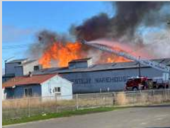
Warehouse Fire in Westley
